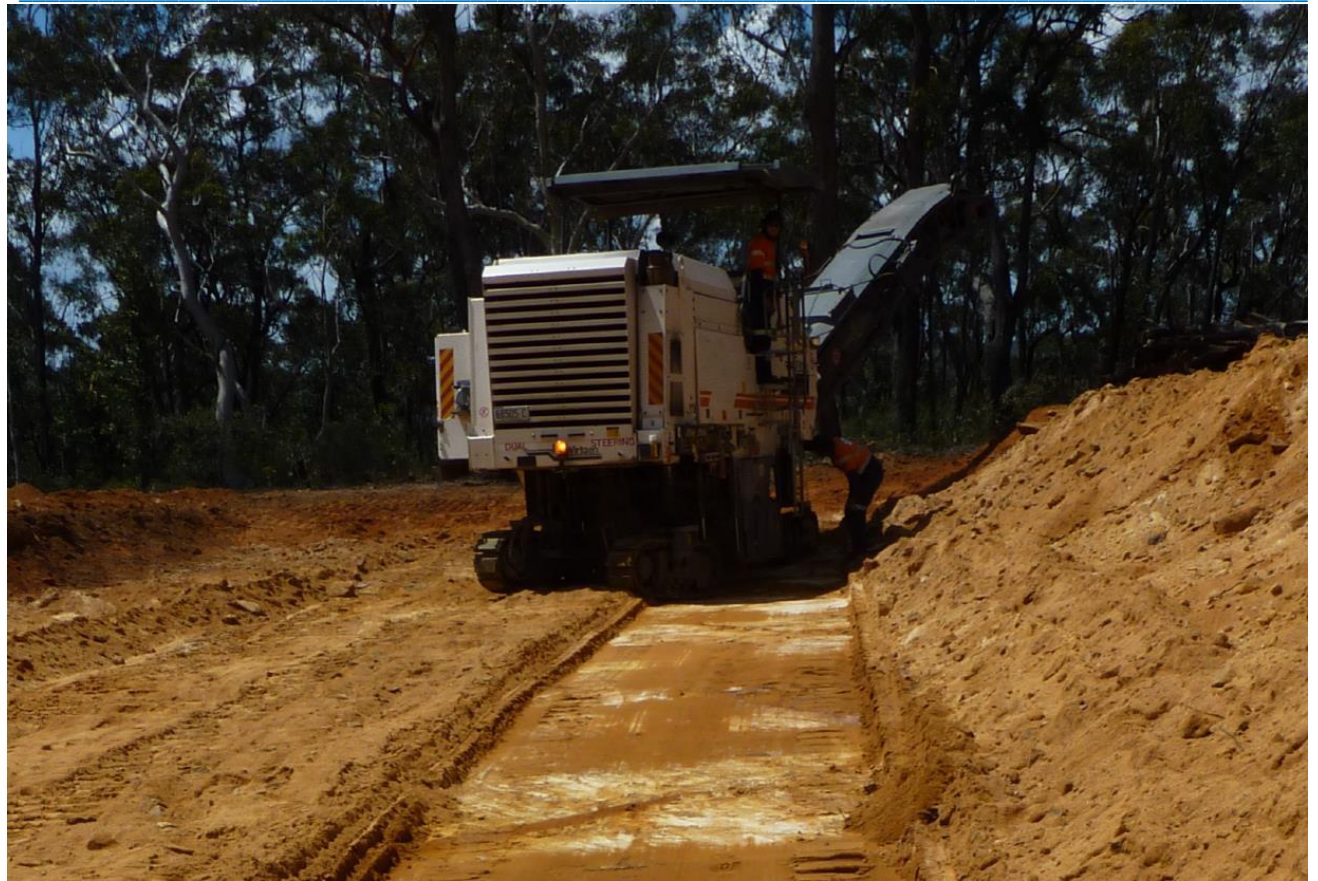
Surface miner in operation - 2009
